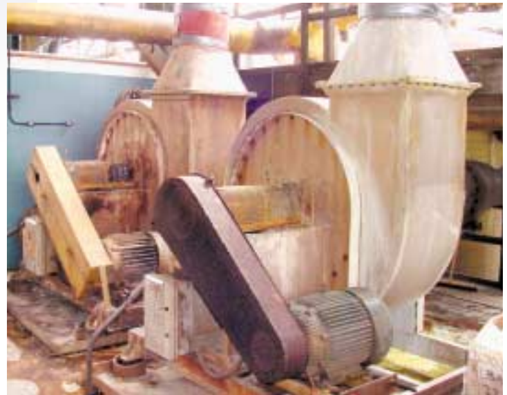
Figure 3. Scrubber blower, with Zirconium or Titanium wheels
